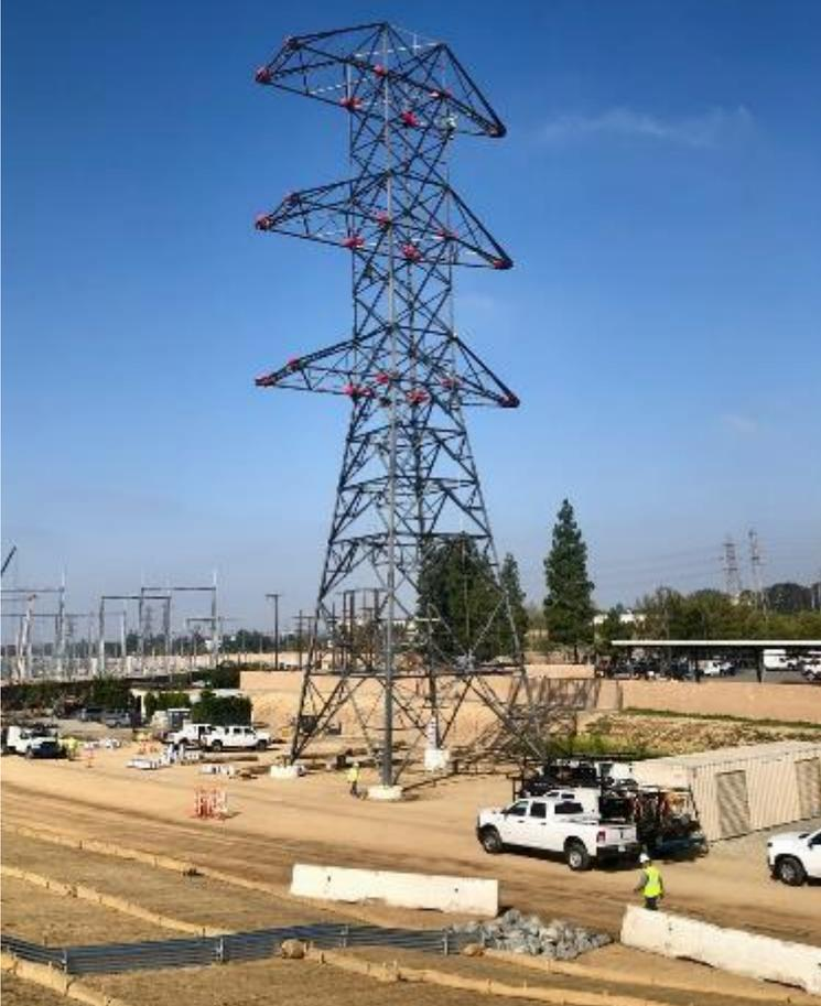
A tall, lattice-work tower under construction at a substation site. The tower is made of steel and has several horizontal cross-arms. It is situated on a dirt area with other construction equipment and vehicles nearby. The sky is clear and blue.              | Photo 1 – A crew was installing raptor exclusion balls to the newly erected lattice work tower north of the construction trailers. Photo facing northwest. |
