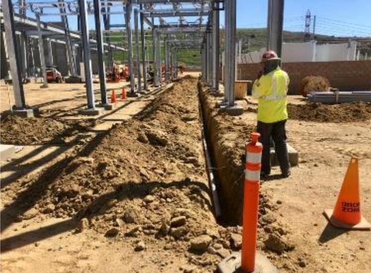
A worker in a yellow safety vest and hard hat is standing next to a trench where conduits are being installed. Orange traffic cones are visible in the foreground. | Photo 8 – Conduit installation. Photo facing south.                                 |
