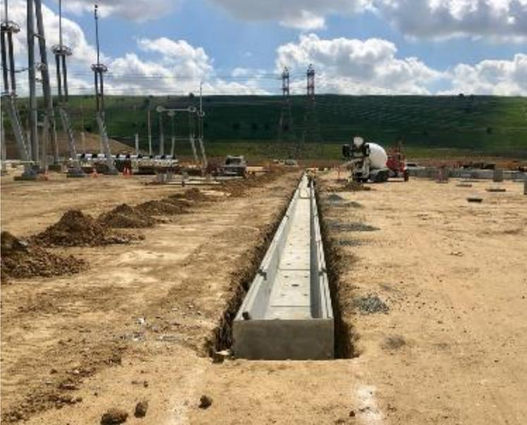
A long, narrow concrete channel for cable trays is being installed in a dirt area. In the background, there are power lines and a concrete mixer truck.             | Photo 7 – Cable tray installation within the Phase 4 work area. Photo facing south. |
